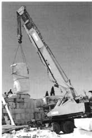
Above, the first drum of the colonnade, a newly-cut one, being put in place. Photo by Anthi Koutsoukou. Right, Chryssanthos Kanellopoulos' restoration of the temple as it was probably actually built.
